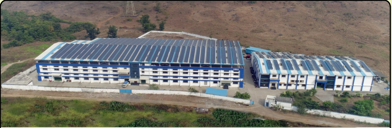
UNIT - 1: Heat Shrink Tube, Moulded Shape, Cable Accessories and PVC Moulding Factory - Palghar
