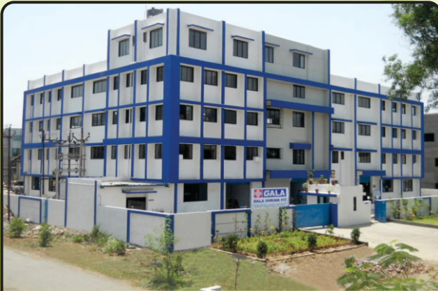
UNIT - 2 Moulded Shape Factory - Surat
